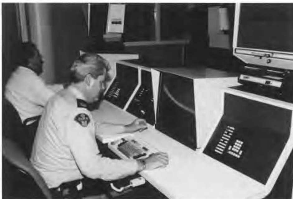
The new Communications Centre at Number 5 District OPP Headquarters in Aurora, Ontario.
