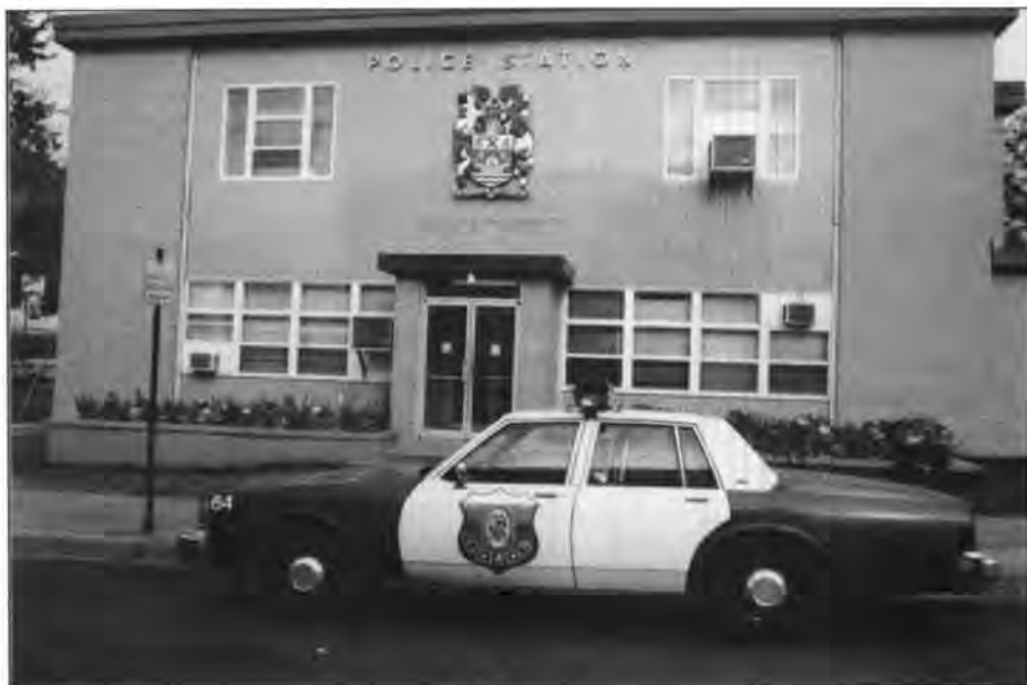
Dartmouth Police Station
