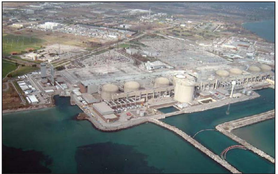
The Pickering nuclear power generation station is one of the higher priority properties included as part of the Durham Regional Police Emergency Management responsibilities.
